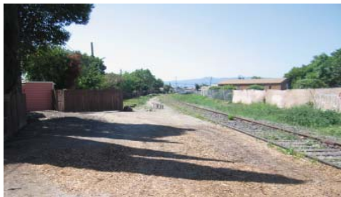
An encroachment into the abandoned railroad right-of-way just south of East San Antonio Street. Graffiti and dumped items are also present.
