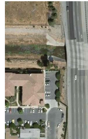
Image of the area proposed for the East Court extension. Image courtesy of Google Earth.
