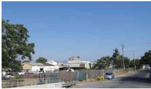
View of the Rail-to-Trail corridor along the east side of Wooster Avenue and just south of Lower Silver Creek (looking south).
