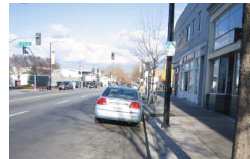
On-street parking along the East Santa Clara Street/Alum Rock Avenue corridor is generally not defined with street paint.
